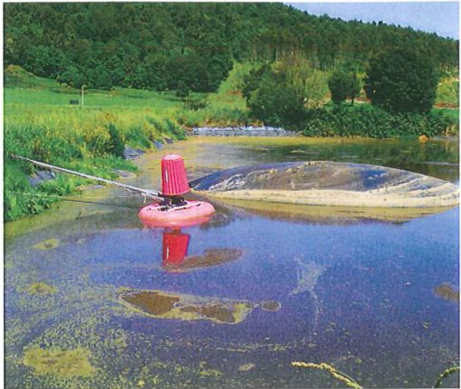
Figure 2: An example of a pond with incorrect gas drainage.
