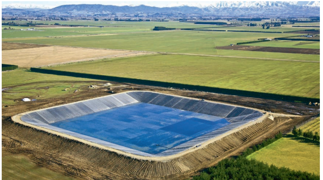
Above: Turley Farms new water storage reservoir in South Canterbury. Below: Laying the liner in Turley Farms new water storage reservoir.
