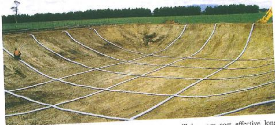
Gas drainage being installed.
