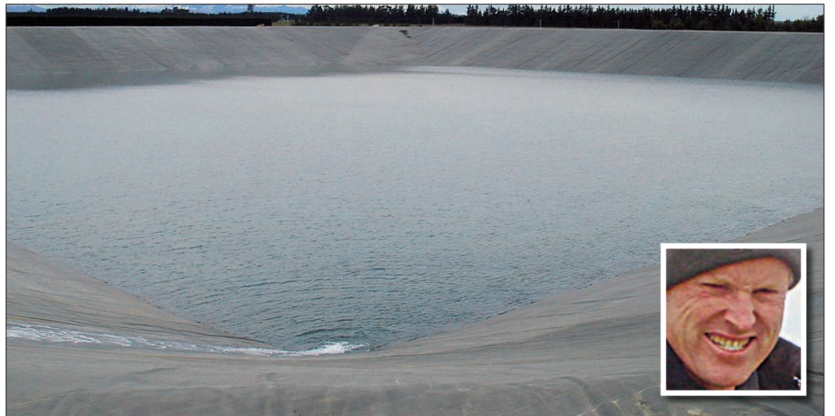
The Turley Farms lined reservoir is now about 25% full. Batter slope is 1:3. Inset, Murray Turley.
