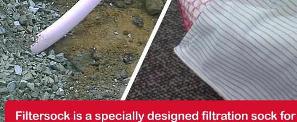
use with perforated drain pipes. Filtersock helps to prevent debris from clogging drainage pipes.
