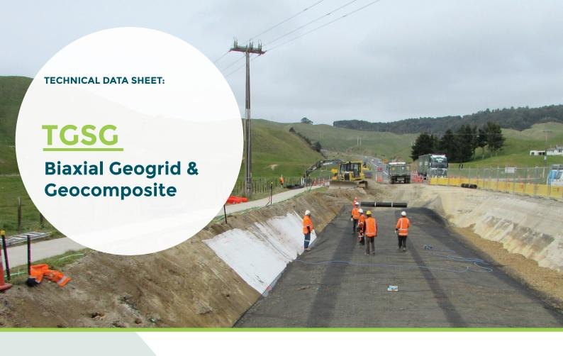
TGSG biaxial geogrids and geocomposites are used for the reinforcement of soils and aggregates in construction of road pavements, hardstands, working platforms and reinforced foundations.
