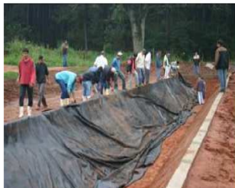
2-EPDM RubberGard installation process
