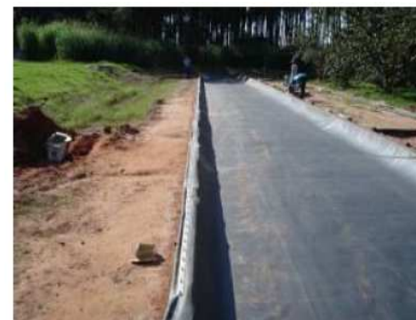
6-Fixation EPDM in the beam
