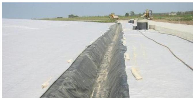
Figure 6. Installation of the peripheral ditch and high protection geotextile
