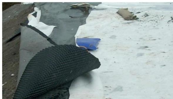
Figure 4. Gas drain geocomposite.
