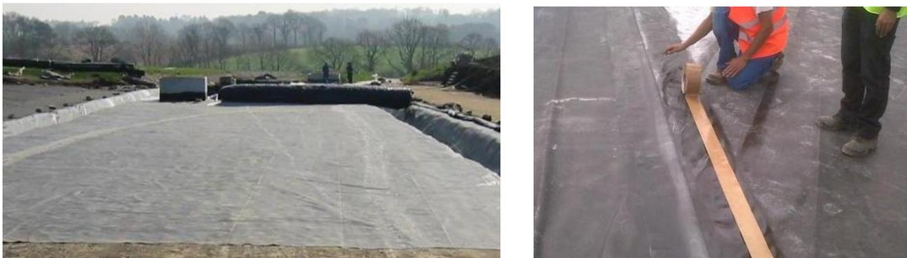
Figure 5. Installation of the EPDM geomembrane. Creating a seal using self-adhesive tape
