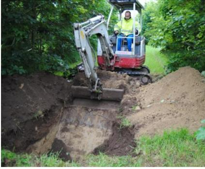
Figure 10. Starting the excavation to take the samples
