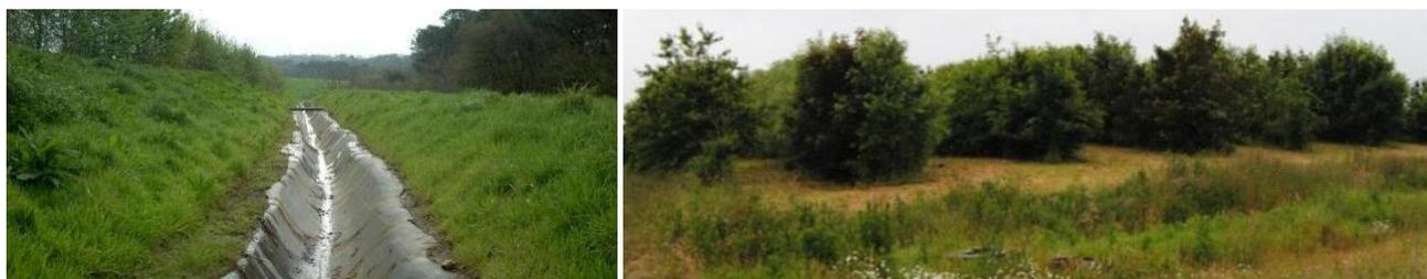
Figure 2. Peripheral ditch at the foot of the mound lined with EPDM geomembrane and current state of the landfill
