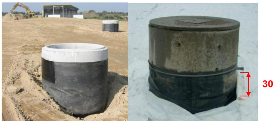
Figure 92. Degassing well before and after the addition of a safety pleat
