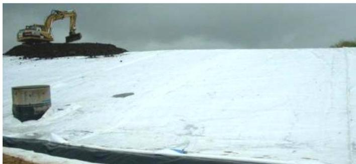
Figure 7. Installation of the soil cover
