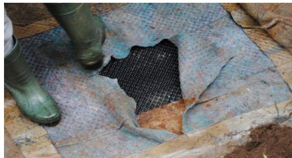
Figure 14. Protective geotextile and gas drainage placed under the geomembrane
