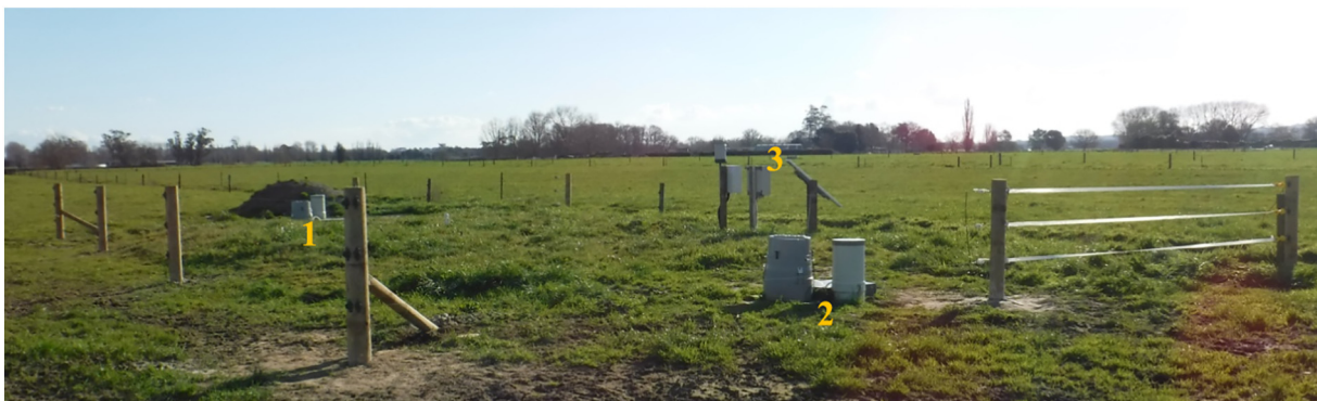
Fig. 3. The completed installation of the Tatuani woodchip bioreactor showing the main components: (1) inlet control structure with auto sampler and stilling well, (2) outlet control structure with auto sampler and stilling well, (3) rain gauge, solar panel, and control panels for the instruments.
