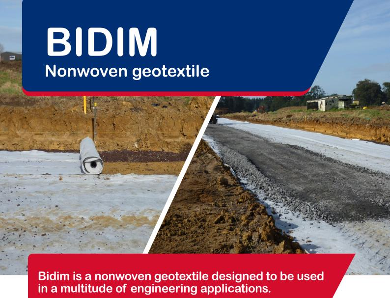
Bidim nonwoven geotextile can be used in; Filtration, Drainage, Separation & Underliner applications. Bidim nonwoven geotextile is manufactured from either Polyester OR Polypropylene staple fibre, then needlepunched for strength. Bidim can be secured to the ground using steel staples, plastic pins, sand bags or rocks. It is recomended that Bidim is overlapped a minimum of 500mm between rolls.
