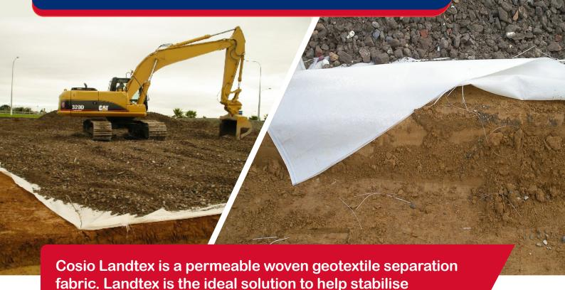
Before laying Landtex, prepare the ground to a reasonable condition, filling ruts or holes with soil or fill. Unroll Landtex over the prepared ground and cover the fabric with hardfill. The hardfill should be spread to a minimum depth of 100mm and at no time should a digger or truck drive onto the uncoverd fabric. Where joins are required, ensure a minimum of 500mm overlap.
